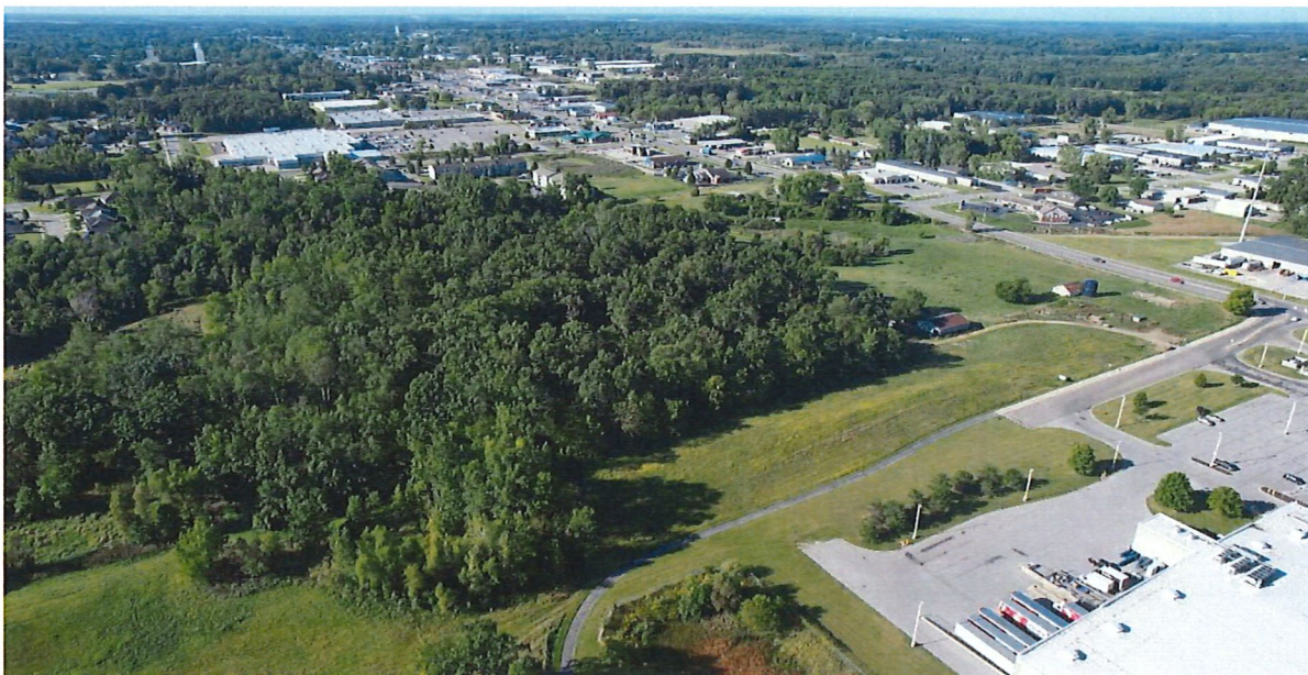
NE Looking SW
