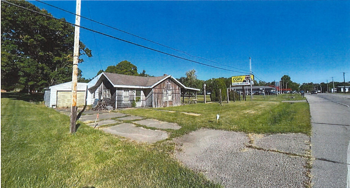
Looking NW from S Wayne St
