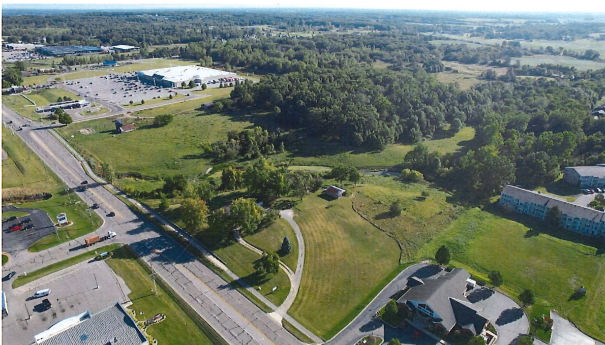
SW Looking NE
